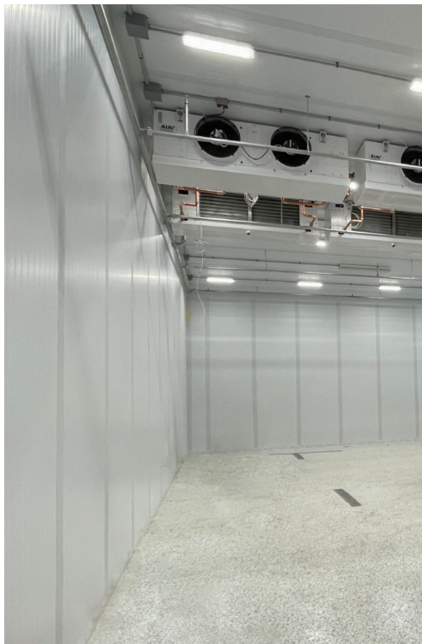
GC Dry Room w/ GC Advantage IMP Gastight Envelope & Temperature/Dehumidification Coils
