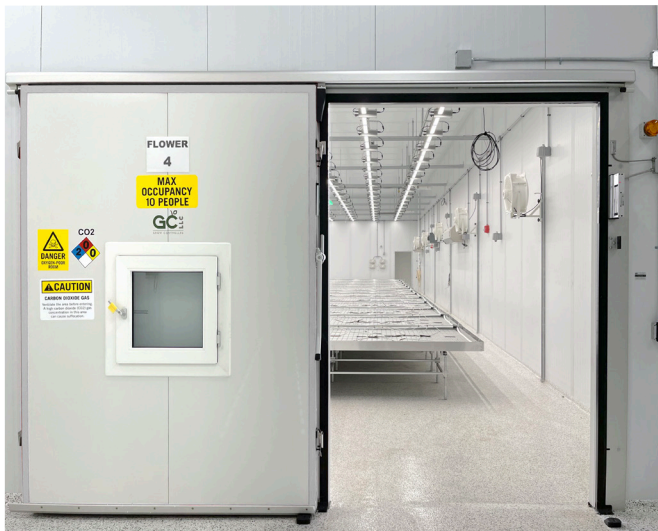
GC PA Grow Room w/ GC Gastight Door & IMP Gastight Envelope
