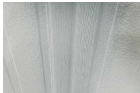
gcfiller seam paint
