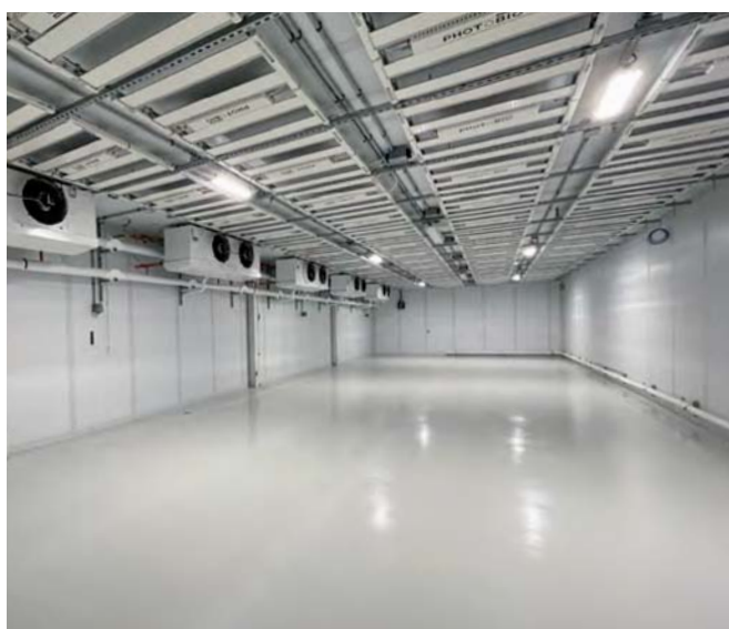
Grow Room Fit-Out with GC IMP & Dehu using Reheat Coils
