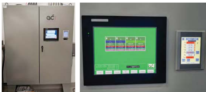
KiloWatch™ Panel with Touchscreens
