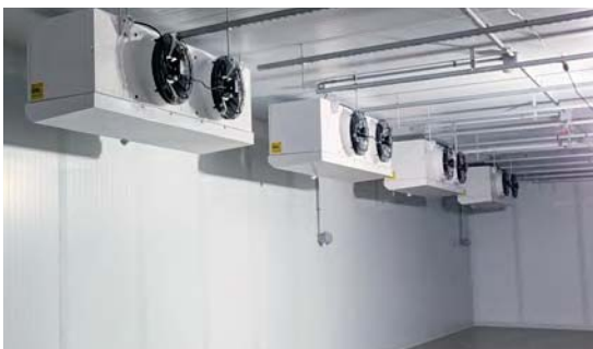
Back-to-Back Coil Arrangement over Aisle in Room
