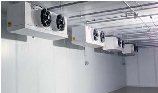
Back-to-Back Coil Arrangement over Aisle in Room
