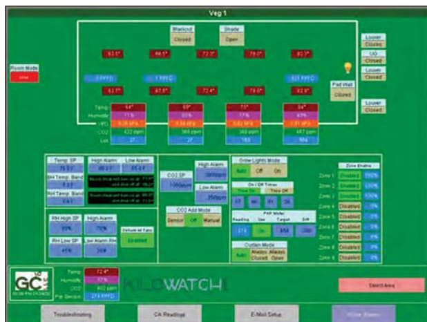
Vegetation Room Overview Screen
