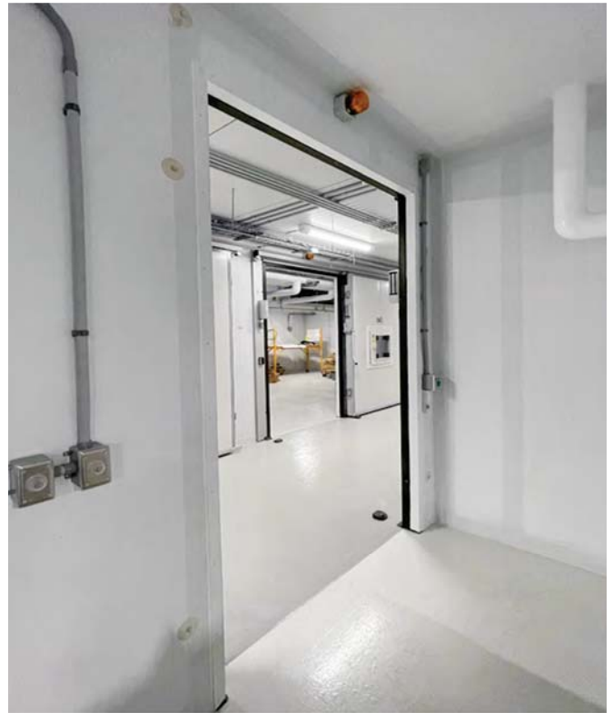
Interior of Grow Room with Growtight Door Installed
