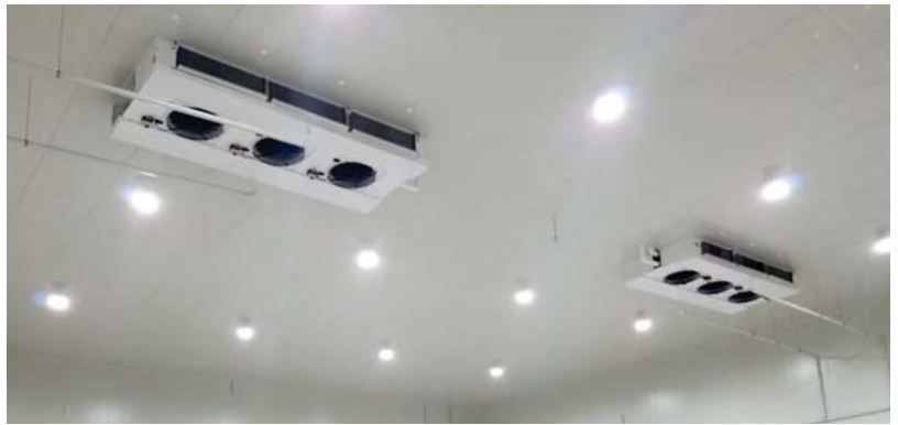
Low Profile V-Flow Dual-Discharge Coils use Less Space and Improve Airflow
