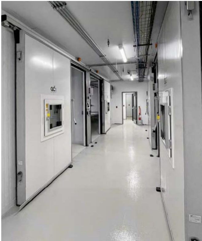
Sliding Growtight Doors in Grow Facility Hallway
