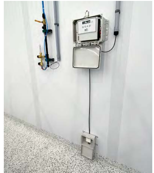
Installed GC QUAD Sensor with Visual LED Alarm Connection
