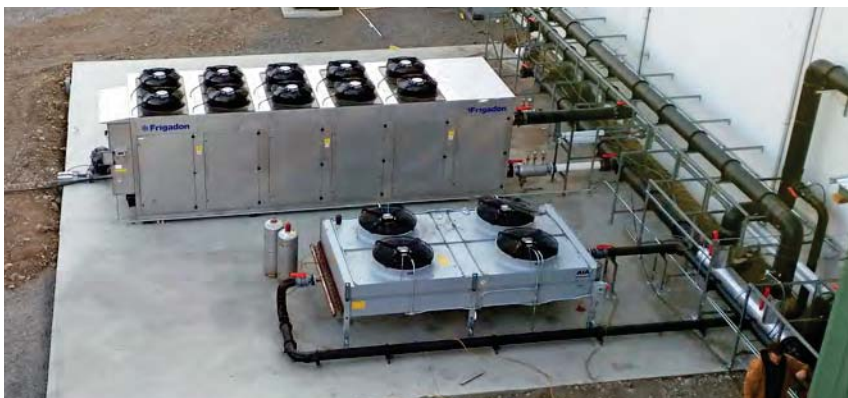
Free Cooler Option using Outdoor Temperatures for Cooling during Winter Months
