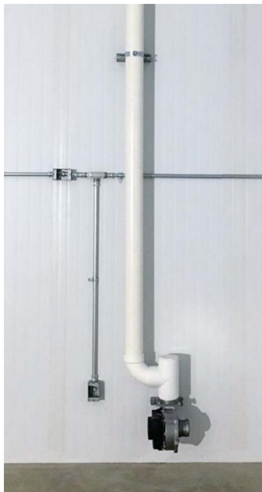
GC CO 2 Safety Valve in Dry/Cure Room
