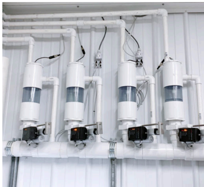
Array of GC Dehu Meters on Individual Drain Line
