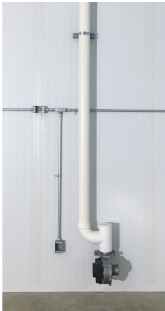
GC CO 2 Safety Valve in Dry/Cure Room
