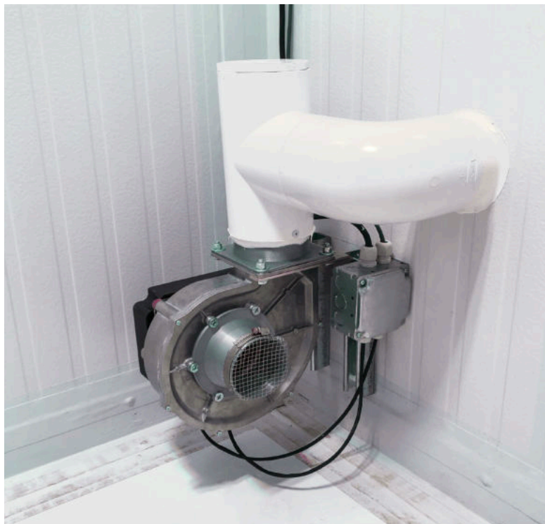
GC Model EC-1 Fresh Air Blower in Grow Room
