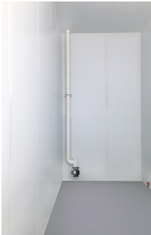
GC SA Holding Room w/ GC Advantage IMP Gastight Envelope
