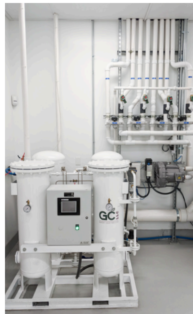
GC Gastight Doors and Nitrogen Generators used to Create GC SA Rooms
