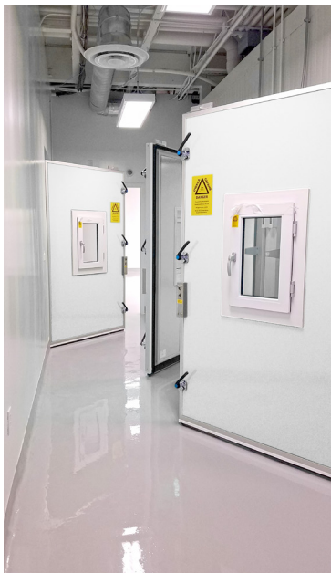
GC Gastight Doors and Nitrogen Generators used to Create GC SA Rooms
