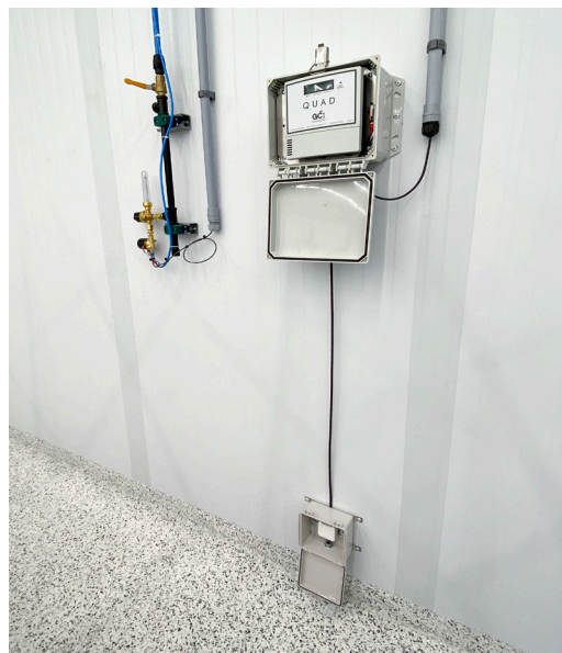
Installed GC QUAD Sensor with Visual LED Alarm Connection
