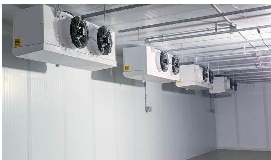
Back-to-Back Coil Arrangement over Aisle in Room
