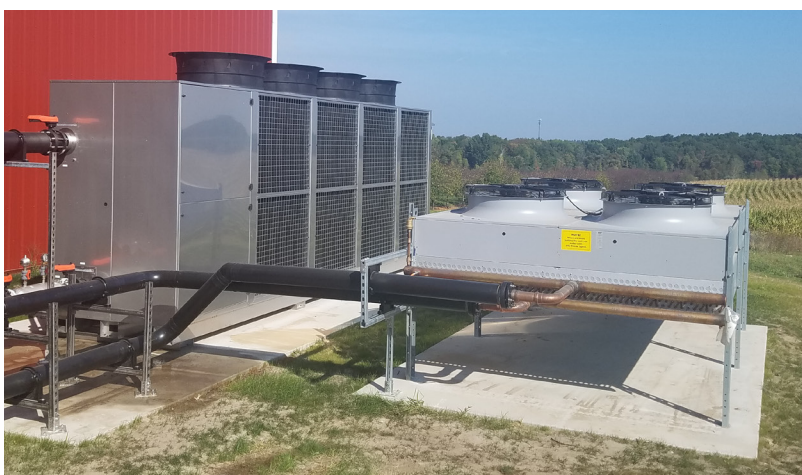
Chiller with Free Cooler Option using Outdoor Temperatures for Cooling
