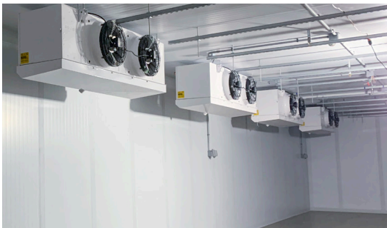
Back-to-Back Coil Arrangement over Aisle in Room
