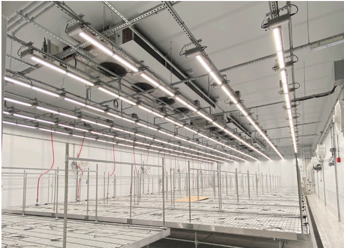
Lights Hang Below Coils for Maximum Canopy Height
