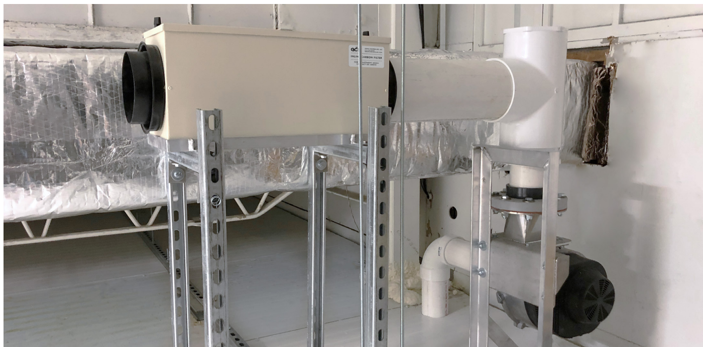
GC ICF Installed on GC Grow Room Exhaust Line
