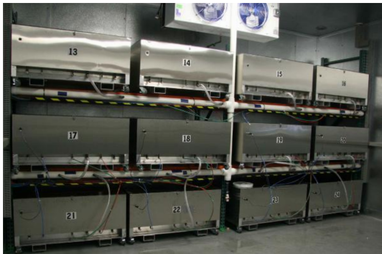
Stacked CūrPod MAX Array in Temperature Controlled Room
